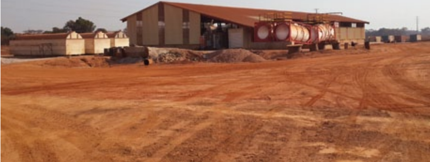
Kansuki Bulk Emulsion Plant. Photo courtesy of AEL Mining Services.
