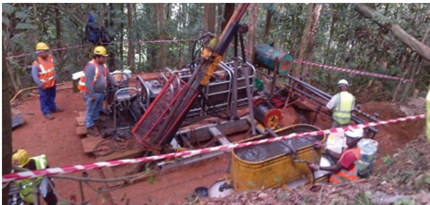
Energold portable series rig in steep forest Central Liberia. Photo courtesy of Energold.
